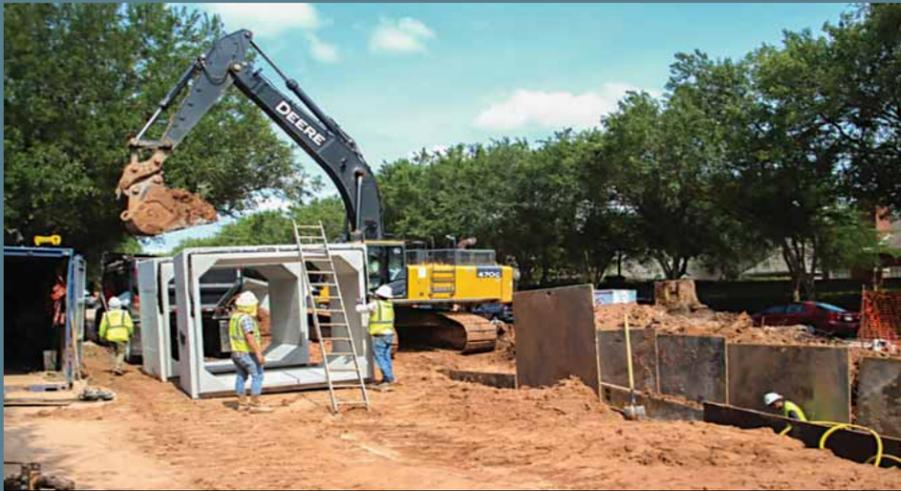
**Drain pipes:** In another project engineered by LAN, these reinforced concrete boxes are being installed in Sugar Land. They are similar to the boxes that will be buried under Walnut Bend Lane to drain rainwater to the flood control ditches before it's ultimately carried to Brays Bayou. (Photo credit: LAN)
