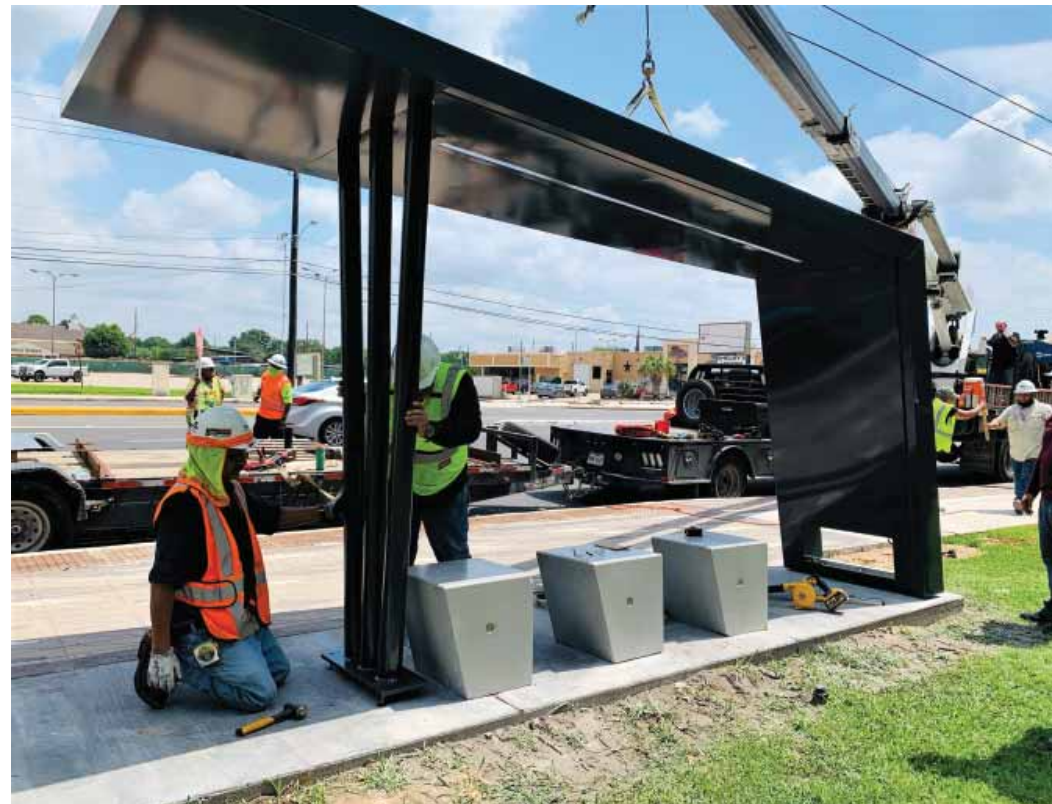
Shady rest: The first of 17 custom bus shelters have been installed on Westheimer Road.
